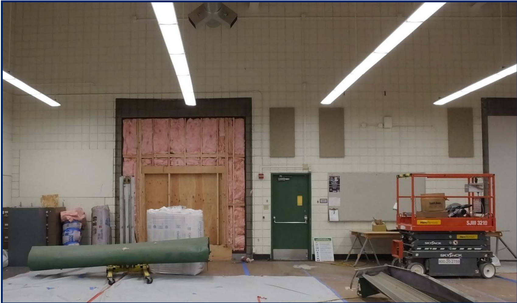
Morrill – Music Room HVAC Upgrade
